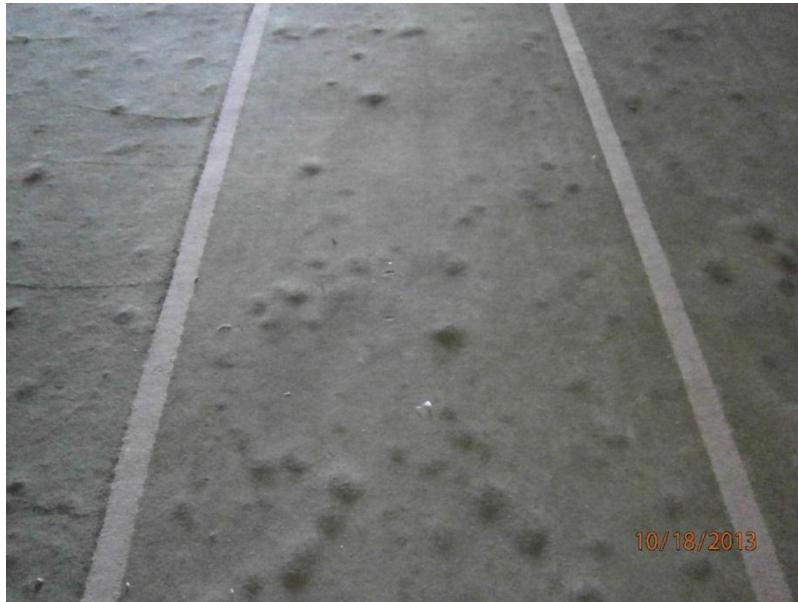
Photograph 2: Damaged synthetic surfacing of tennis court comprising numerous subsurface protrusions.
